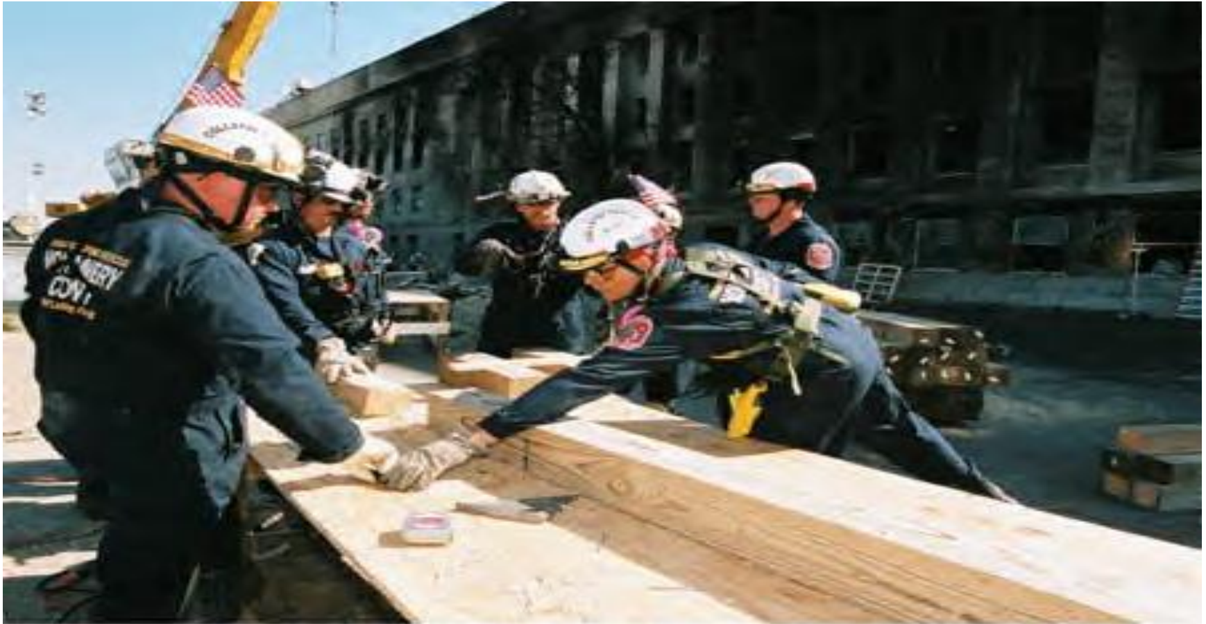
Arlington, VA, September 13, 2001 -- Urban Search and Rescue crews from Montgomery County work to build columns to support the collapsed structure at the crash site following Tuesday's attack.
